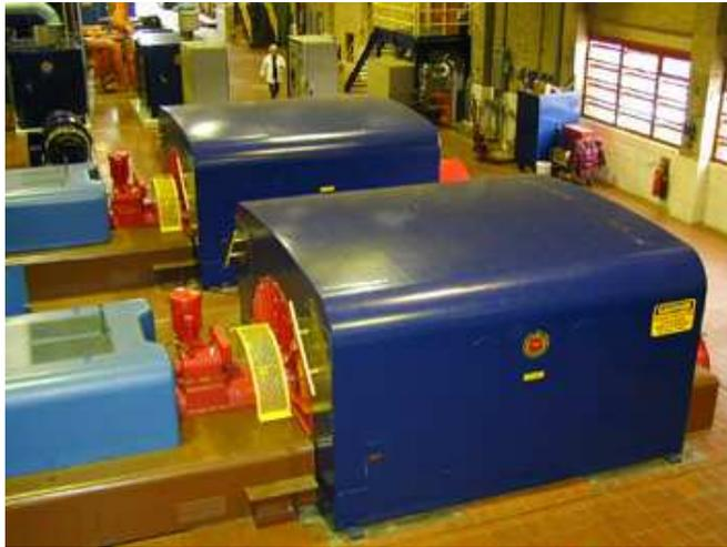
**Figure 7:** the electric generator is a direct application of Faraday's Law of electromagnetic induction. Here are two synchronous generators on the floor of a generation plant.
